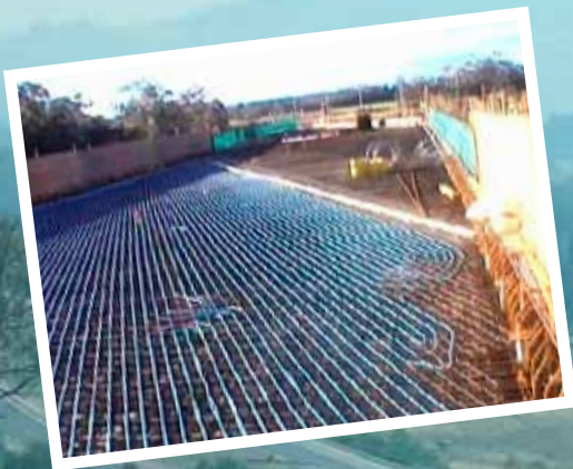
The bridge deck heating coils were installed during construction
